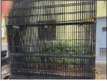
NO CLIMB FENCE
